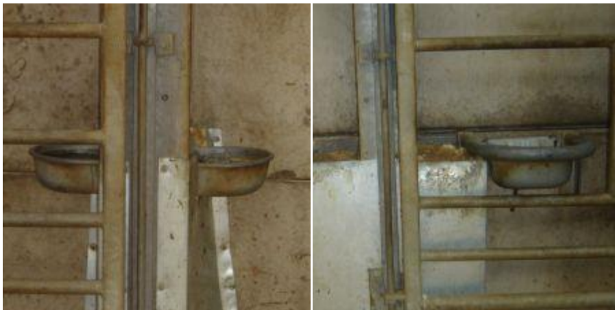
Figure 17 - Drinker blocked by gate Figure 18 - Adapted gate
